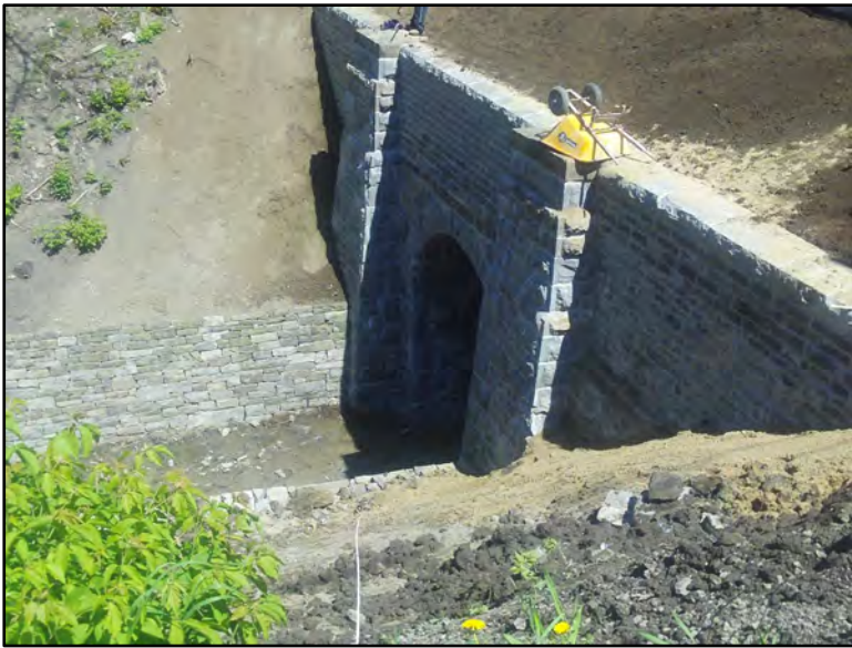
North Portal of the Tunnel
