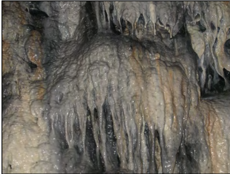
Cave-Like Environment Inside Tunnel
