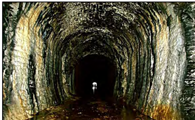
Interior of the Tunnel
