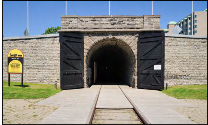
Exterior View of Tunnel, South End, Looking North
