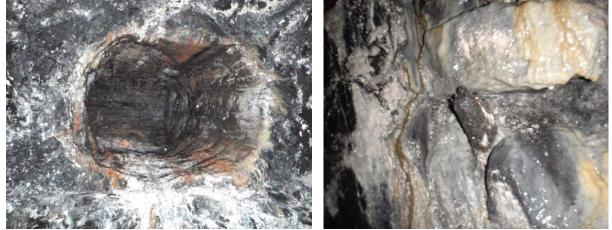
(Left) Rock Hoisting Chimney at 230m. (Right) Corroded iron bar holding brickwork at 295m
