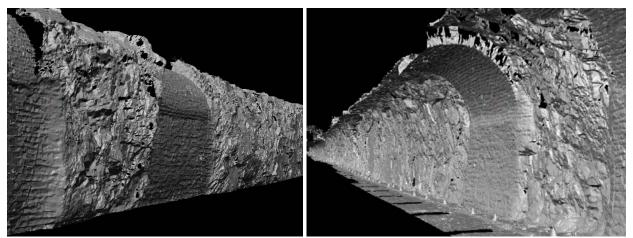
Lidar meshed models of brick/rock interface at +165m. Left image is an outside view, right image is an inside view. The 2D model can be viewed from anywhere in space.
